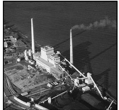
Hydrothane racks have been installed in fossil plants across the USA.
